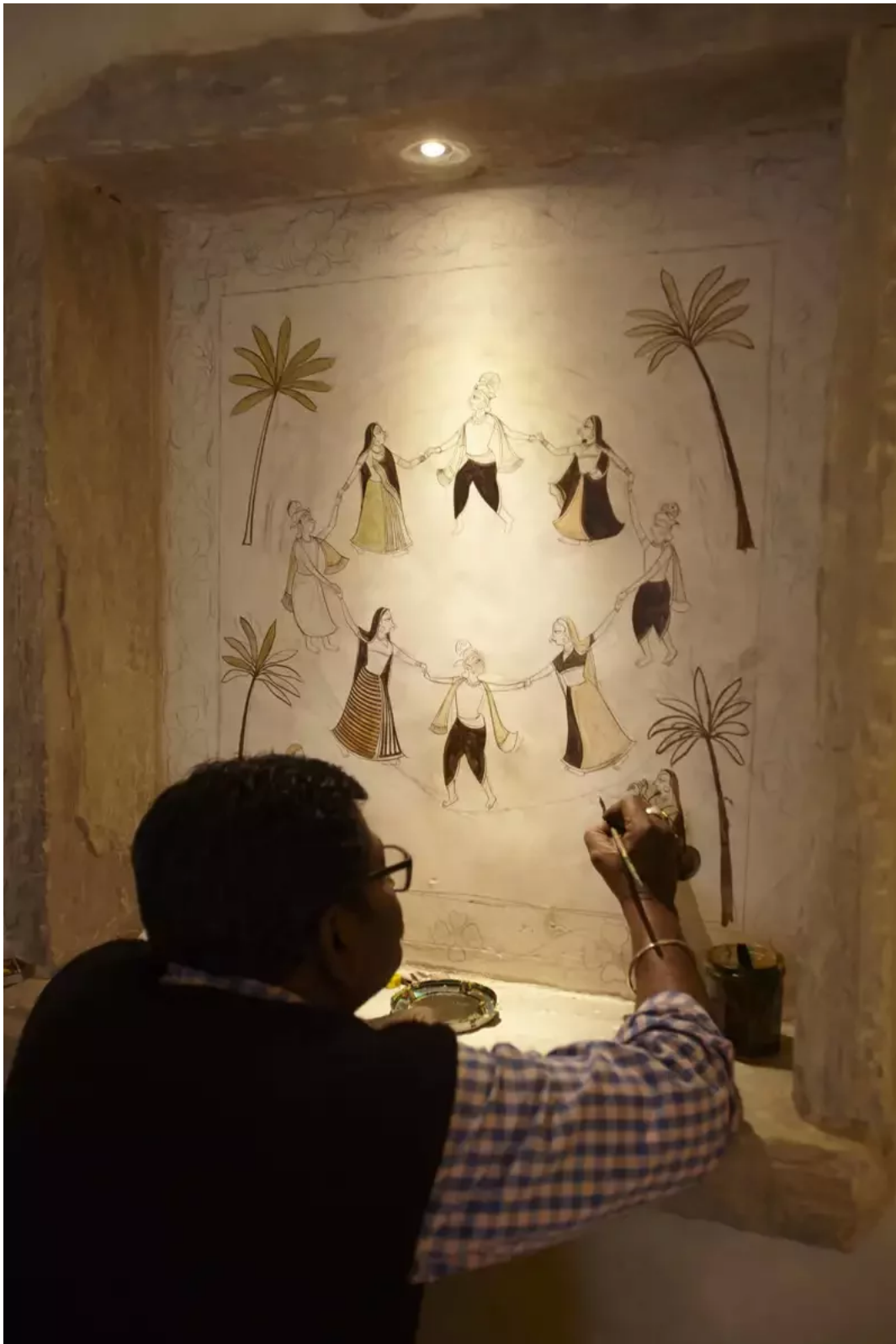
Craftsmen are repairing with unparalleled craftsmanship. Picture / Provided by Kuanting Aesthetics
